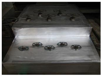
Pre covered to mineral wool flat slab insulation, installed costs compared to metal cladding were 56%.
